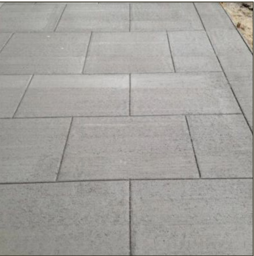
Concrete Decorative Jointing
